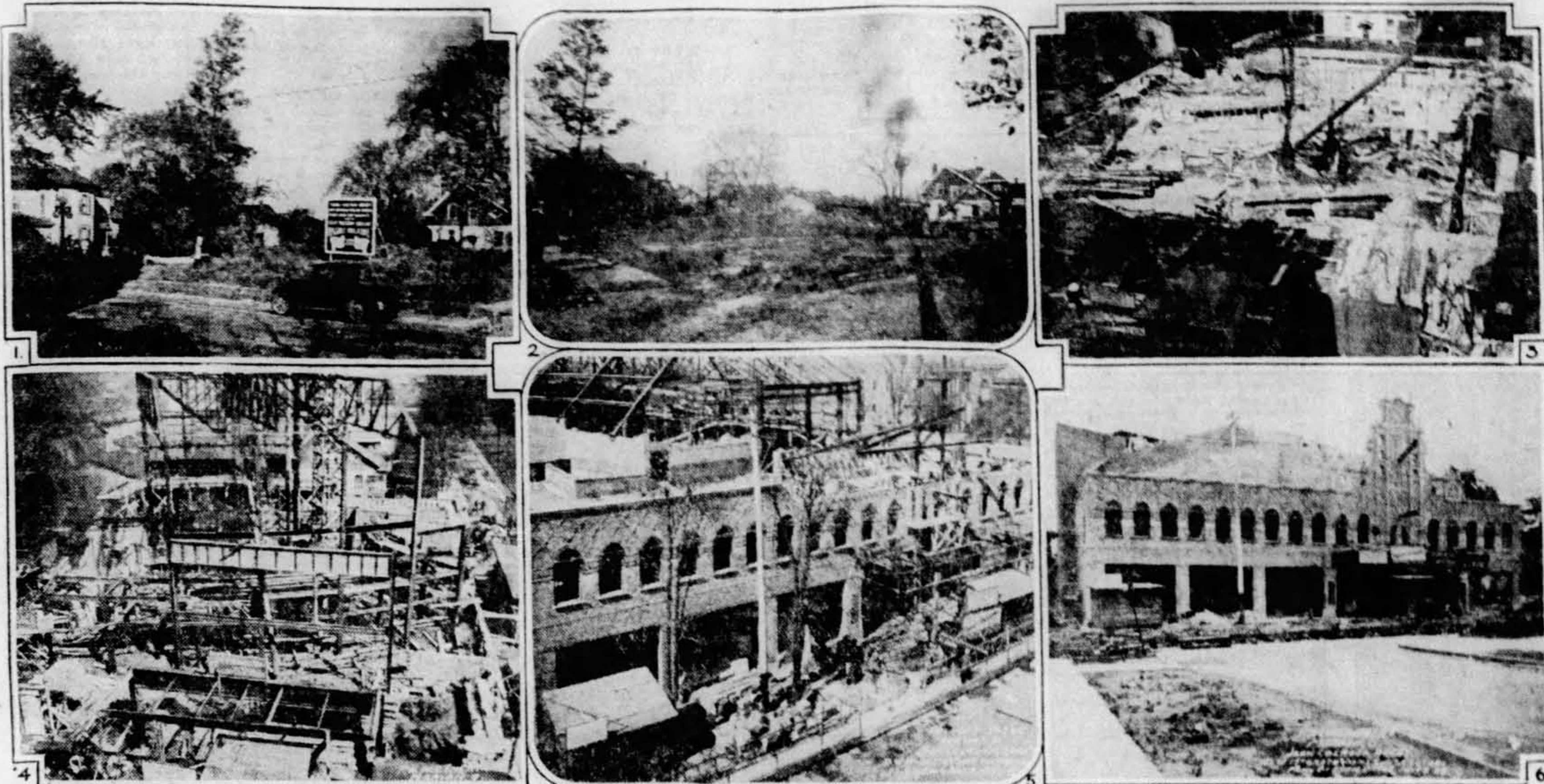
Above are views of the new Palace theater, from the day the sign announcing the house was erected up to June 8. Upper row, left to right, shows: the original site, first excavation work and first foundation work on March 1. Lower row, left to right, shows: the appearance of the site on April 2, the building one month later, May 1, and the structure as it took its final form on June 8.
