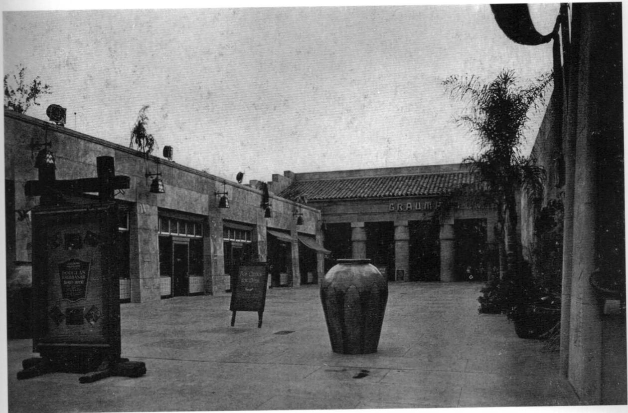
GRAUMAN'S EGYPTIAN THEATRE, HOLLYWOOD, CAL. MEYER & HOLLER, ARCHITECTS.
