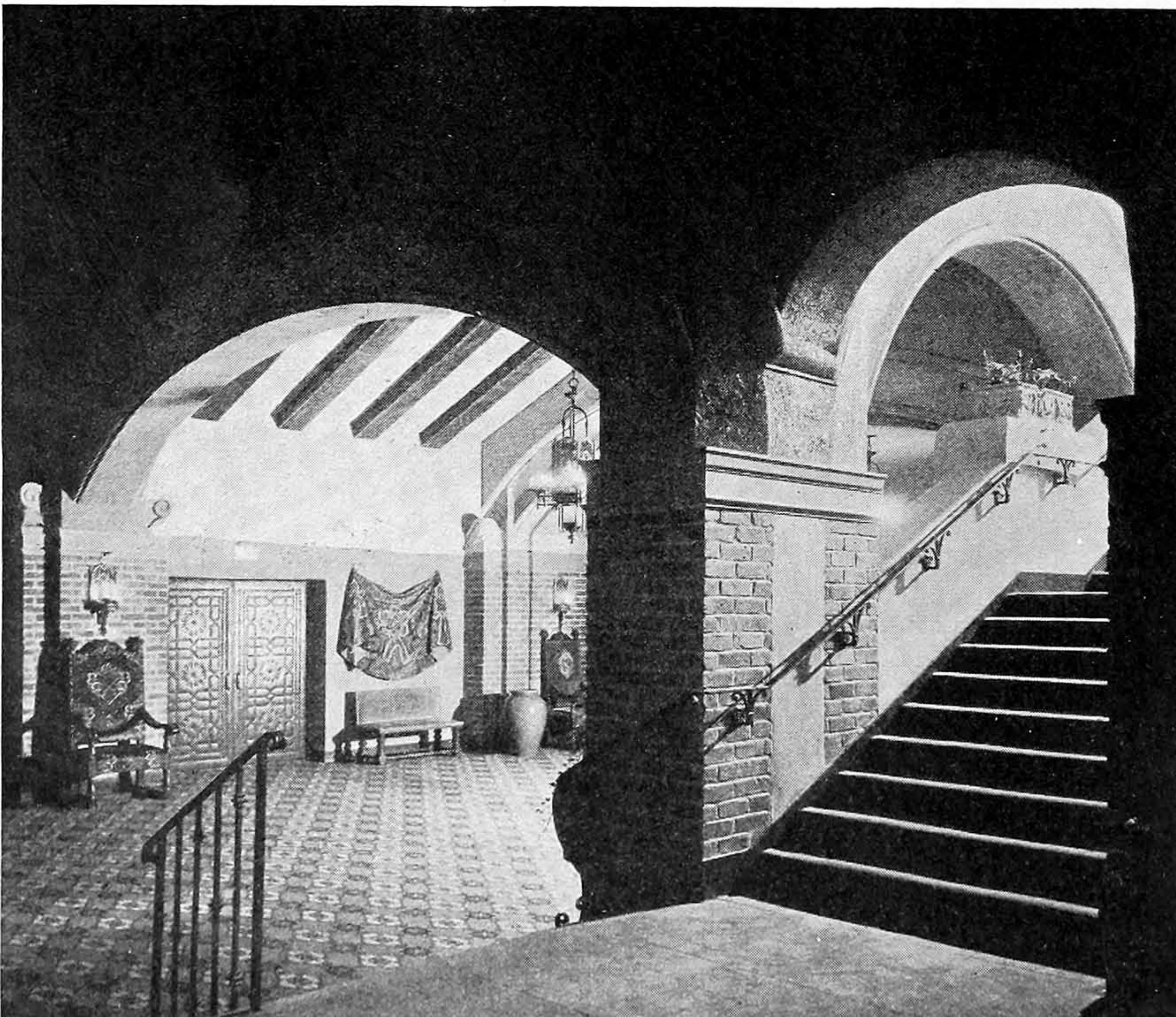
Looking into the lobby from the entrance stair landing.
