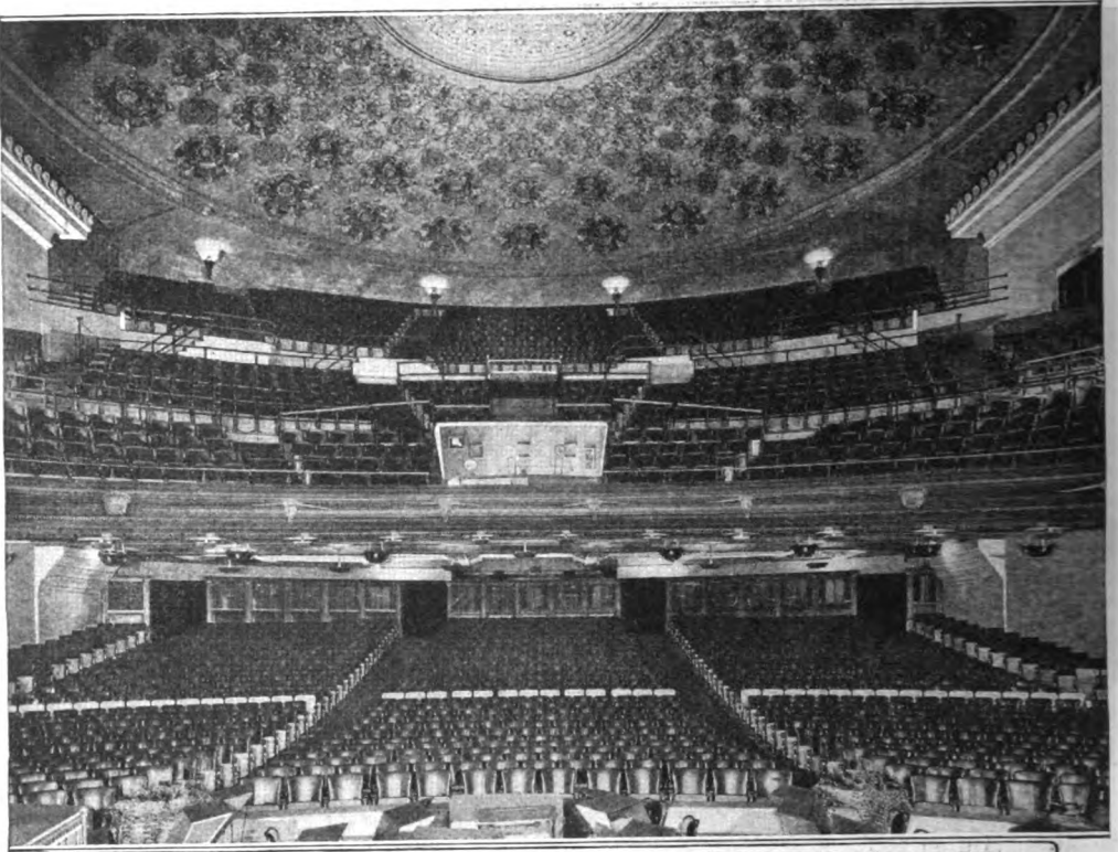
Interior of Los Angeles' Million-Dollar Theater as Seen from the Stage: There Are No Pillars under the Balcony to Obstruct the View of Persons Seated on the Main Floor. In the Center of the Picture may be Seen the Projecting Room. Visible at the Top Is the Gorgeous Jeweled Dome, Which Appears to Those Sitting under It to be Suspended in the Air.
