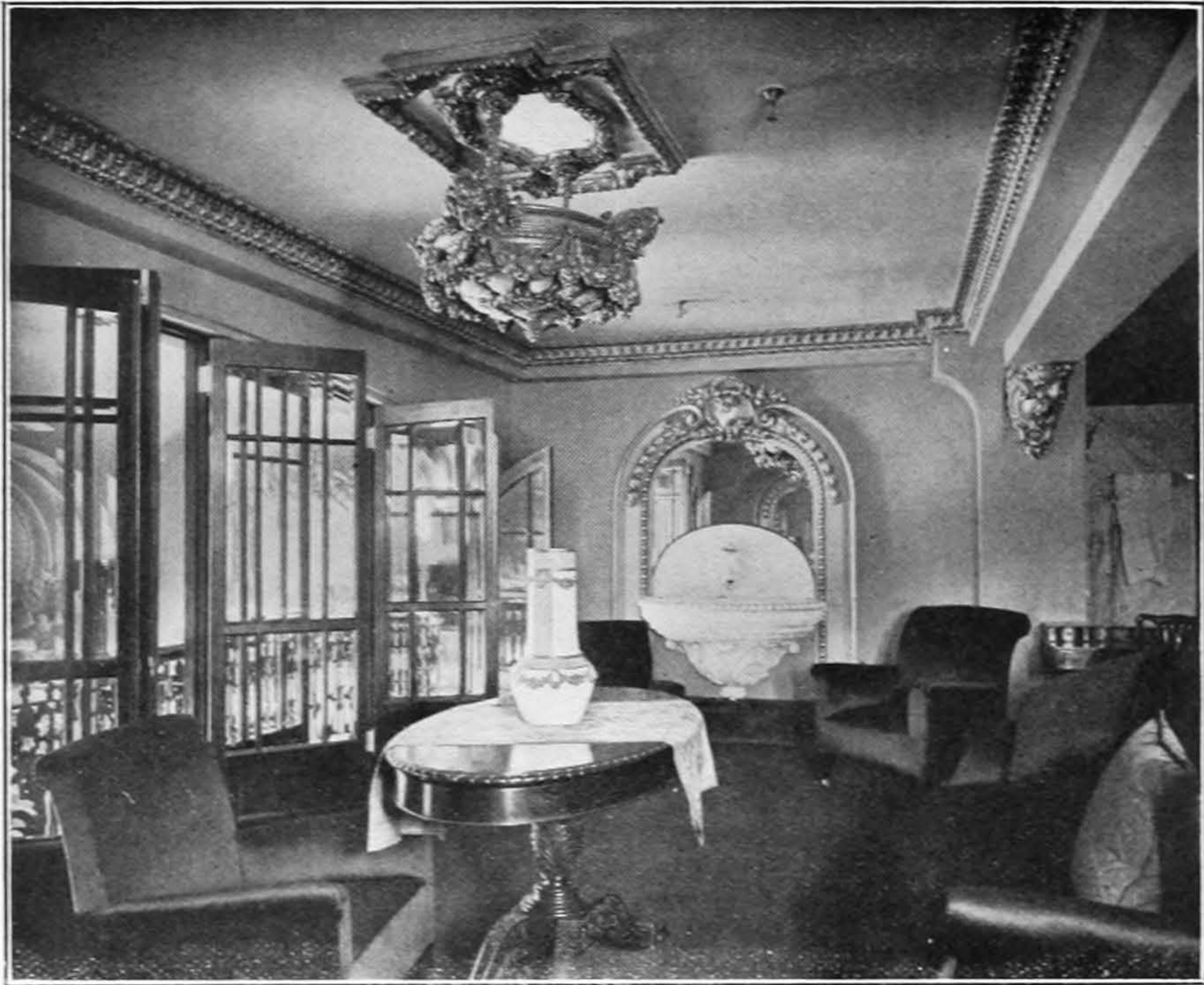
Ladies' Parlor, Orpheum Theater, Los Angeles Plumbing by James W. Hellman, Los Angeles
