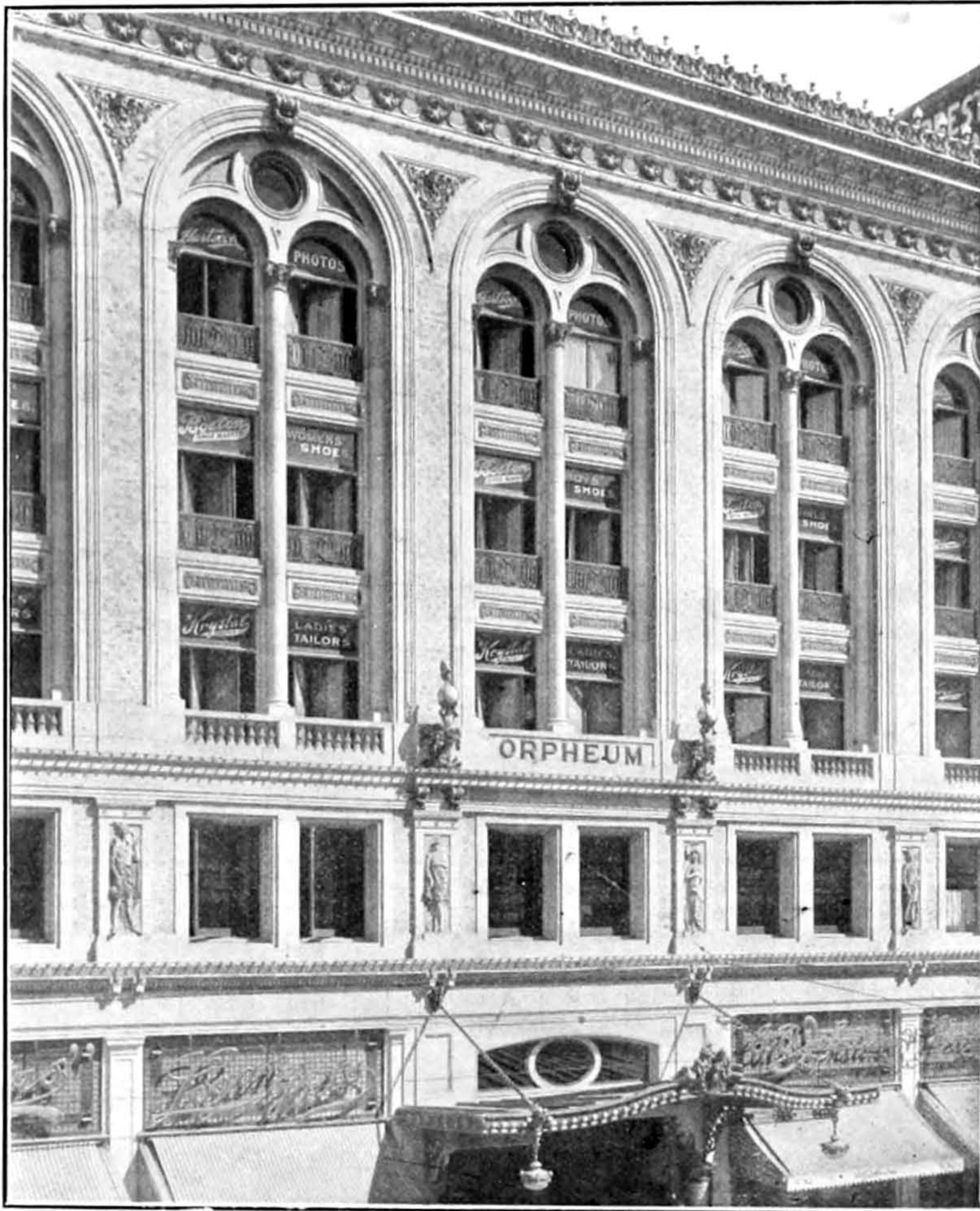
Detail of Broadway Front, Orpheum Theater, Los Angeles Riverside Portland Cement Used
