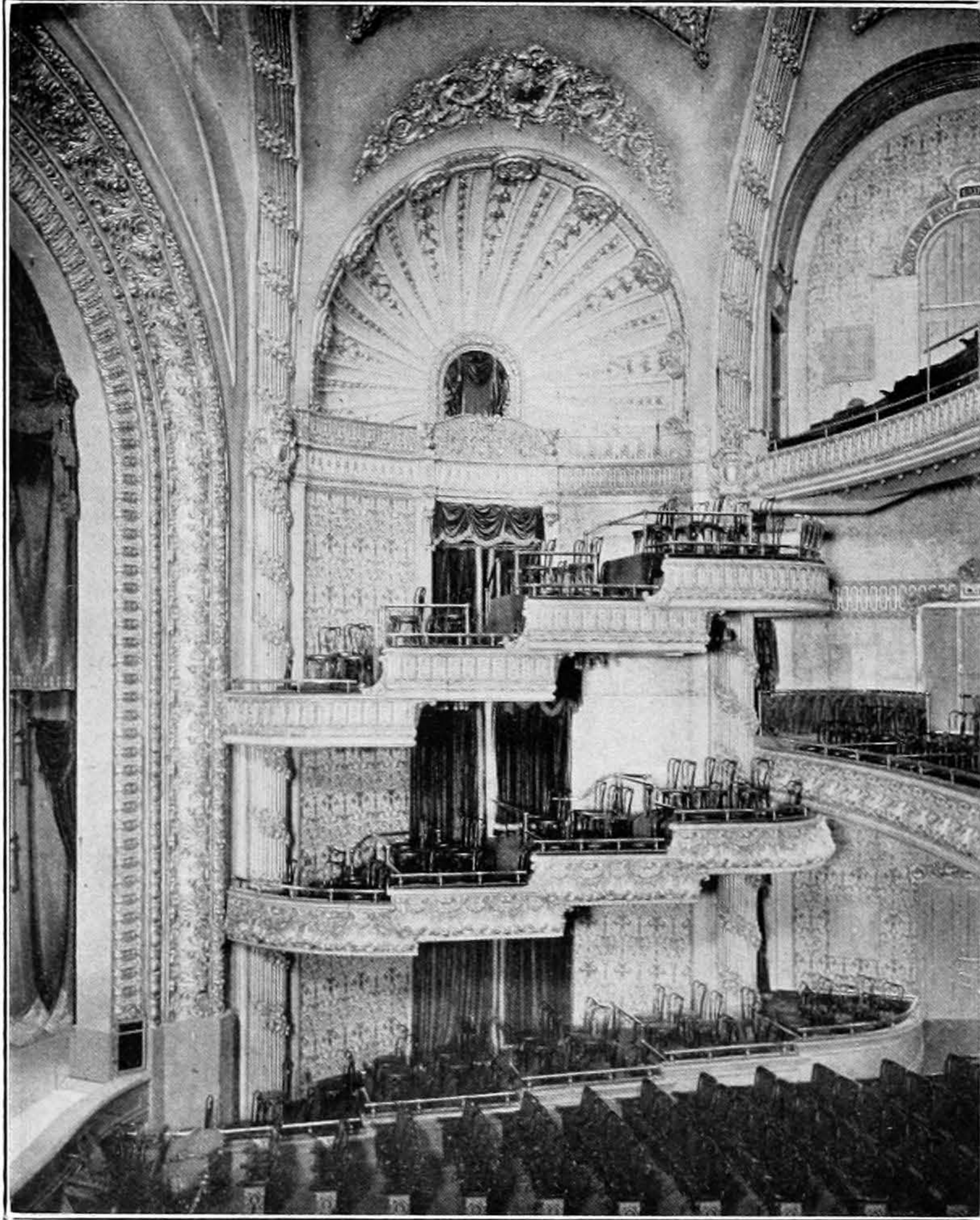
Interior Orpheum Theater, Los Angeles, Showing Arrangement of Boxes Steam Heating and Ventilating Installed by Eugene Murray, Los Angeles G. Albert Lansburgh, Architect
