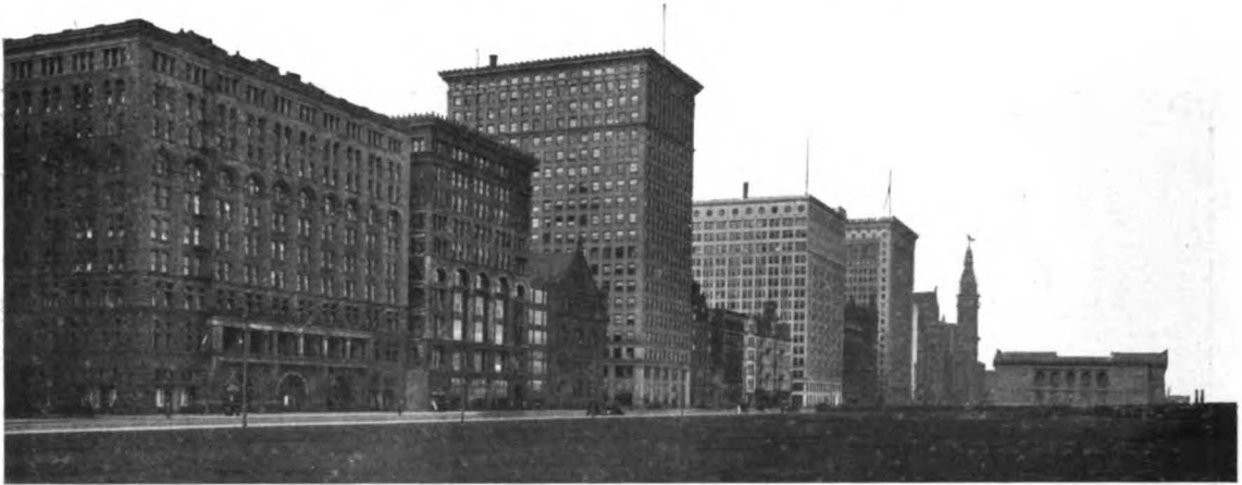
PART OF THE LAKE FRONT, CHICAGO. THE FINE ARTS BUILDING IS THE SECOND FROM THE LEFT, THE ART INSTITUTE ON THE EXTREME RIGHT
