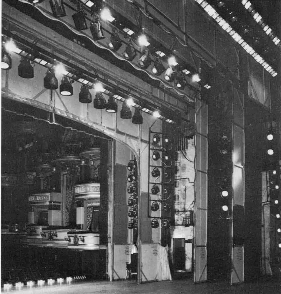
(above) Lighting layout for Carousel 1950 showing Patt. 56 acting area floods overhead. (below) A Chorus Line at Drury Lane today, showing temporary follow spot room top left; sound control front of the dress circle; additional lighting positions in the upper circle and at the proscenium.
