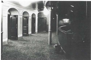
First circle crush area which was opened up to link to the auditorium and bars.
